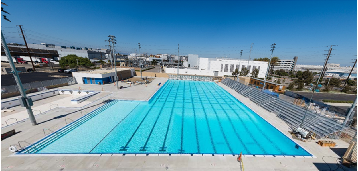
2018 – City of El Segundo-Wiseburn Unified School District Aquatics Center
